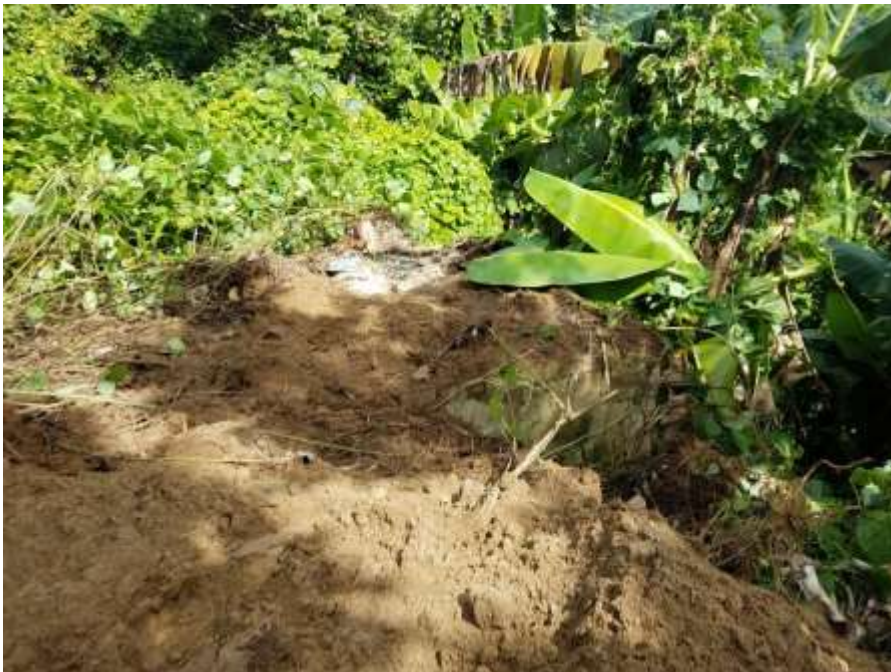
Photograph 12: Empty septic tank system.
