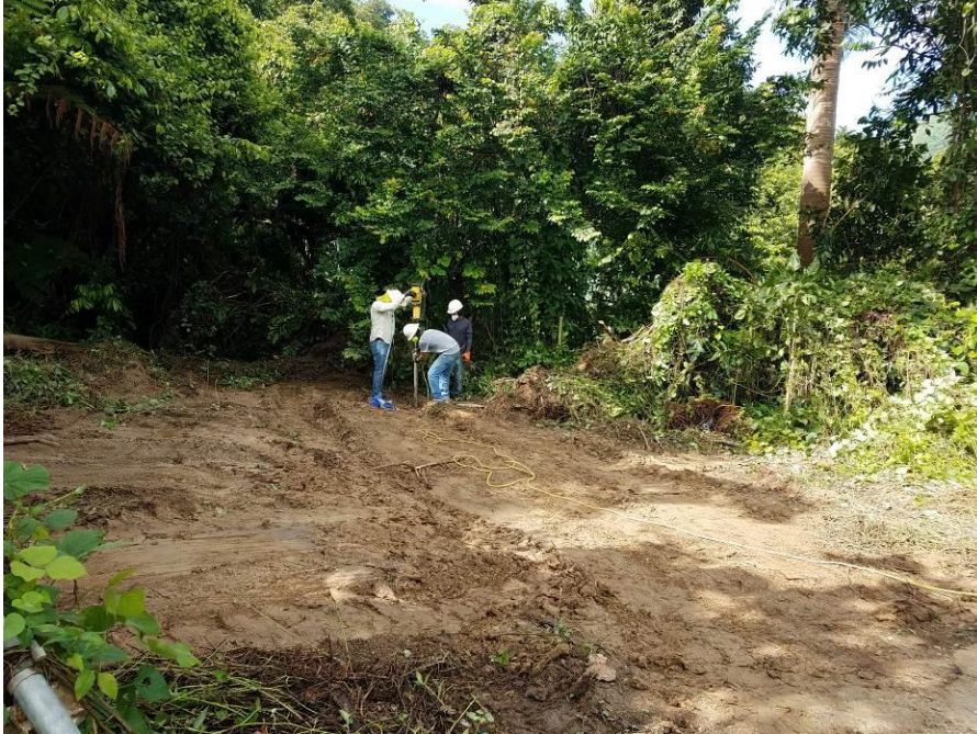
Photograph 1: Soil boring drilling at SB-1.
