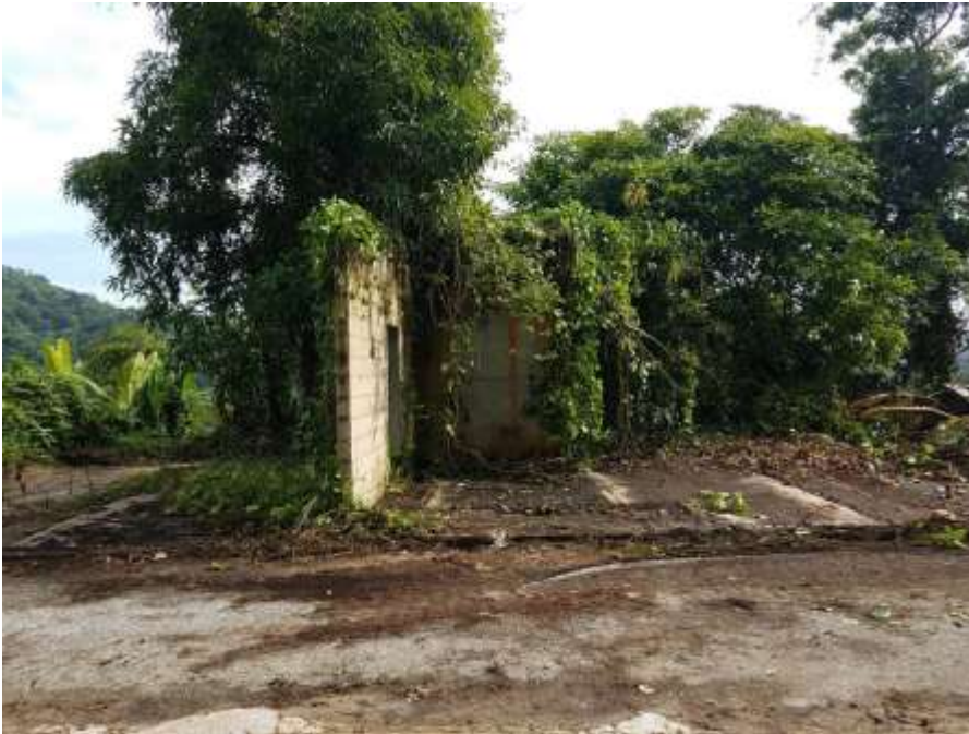
Photograph 10: Partial view of former mechanical shop.
