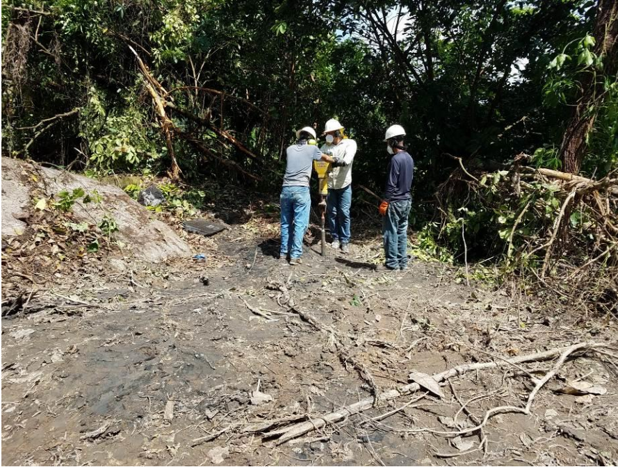
Photograph 3: Soil boring drilling at SB-6.
