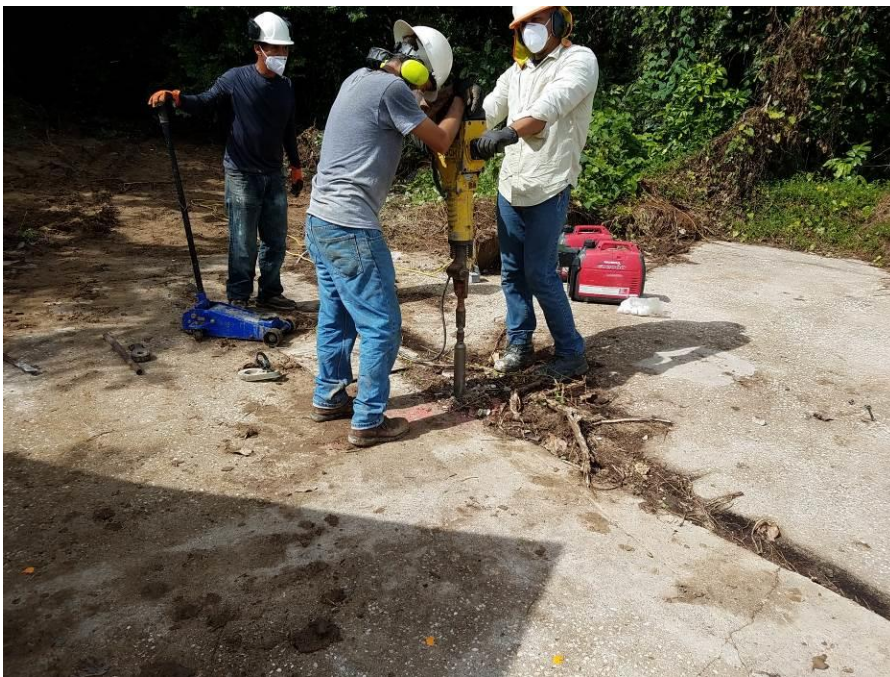
Photograph 2: Soil boring drilling at SB-2.
