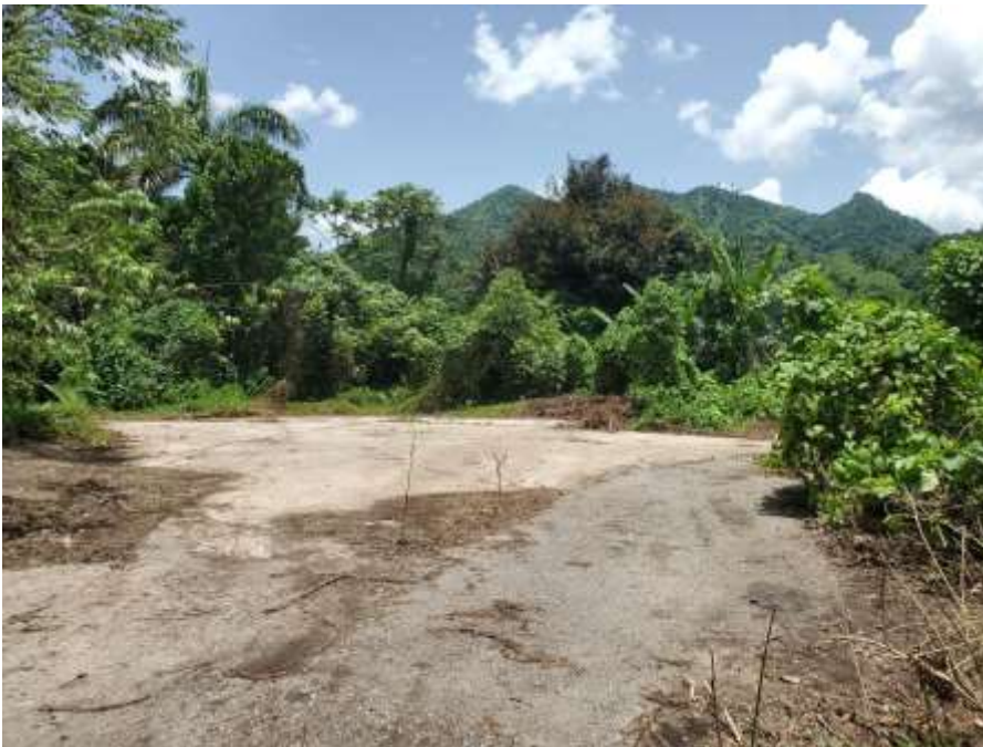
Photograph 8: Partial view of paved concrete slab floor the former residential and mechanical shop.
