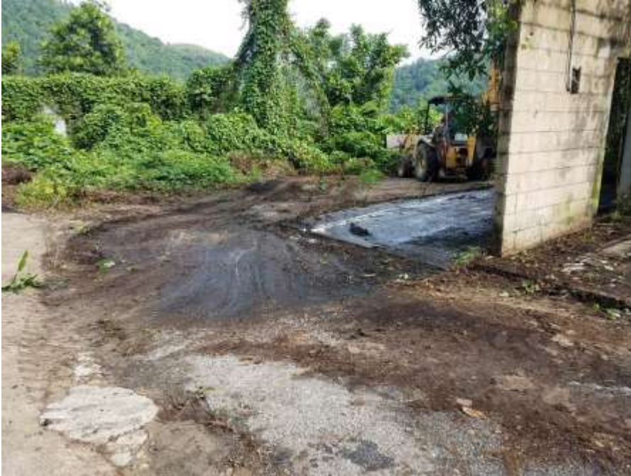
Photograph 13: Stained ground surface.
