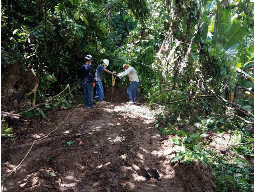
Photograph 5: Soil boring drilling at SB-7 (BKG).
